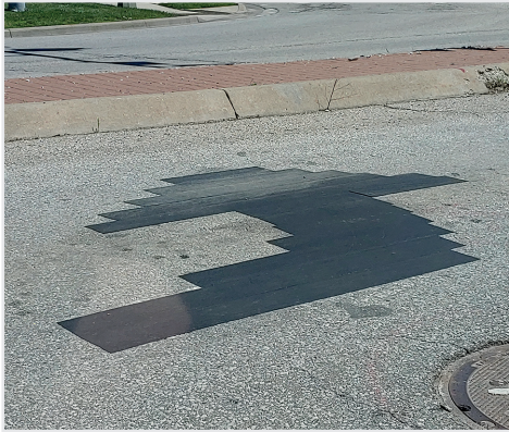
A turn lane arrow grayed out during road construction by overlaying the white arrow with black.
