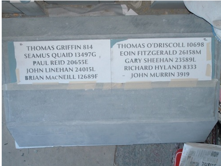
The stonecutter placed the full-sized printed sheets onto the stone before carving.
