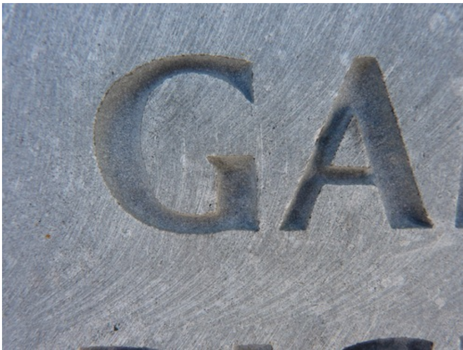
The “G” and “A” carved in limestone without any infill color. The “G” has lost some of its elegance.
