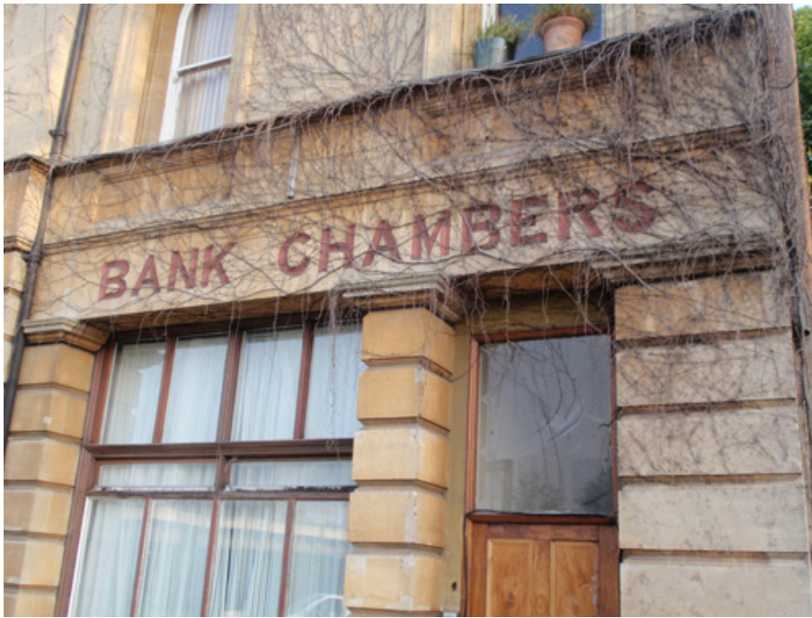
Bank Chambers in Haringey, north London, suggests solidity with its bold square sans serif. It may have been made by pressing wood pattern letters into wet cement.
