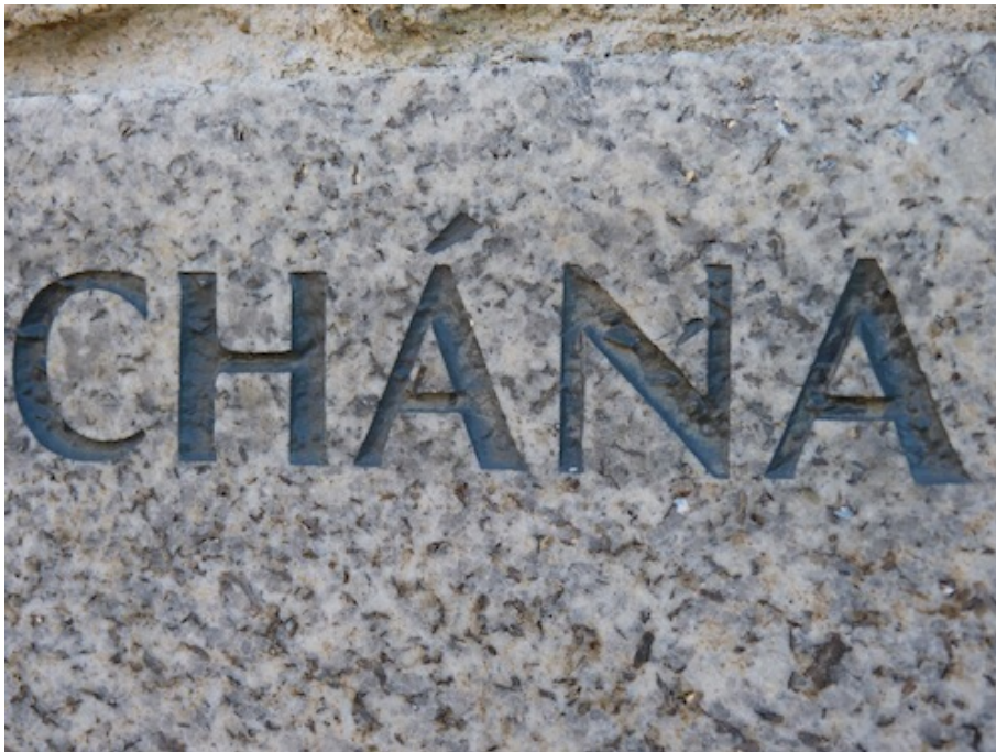
A detail of the carved lettering in speckled granite, with dark-gray infill.
